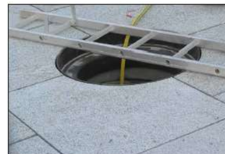
MONTERT RAMME BELEGG
